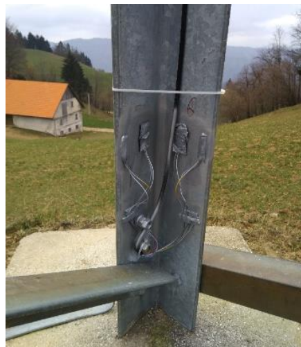
Figure 3: Adhesive strain gauges at the location of the measured residual stresses on the L profile [20].
