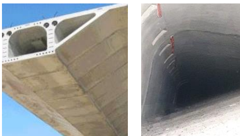
Figure 1: A confined space for indoor inspection: box girder bridge and detail of the cross-section.
